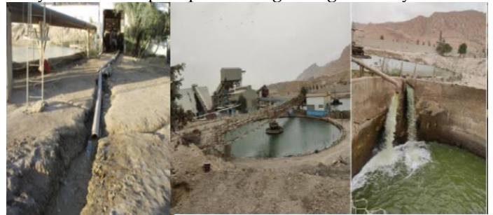
Fig.5. Liquid effluent discharge from the phosphate desliming process
