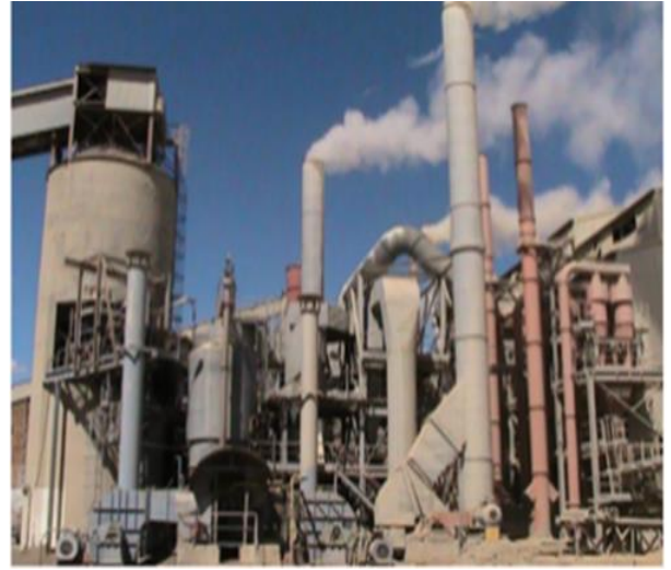
Fig.3. View of the processing plant.
